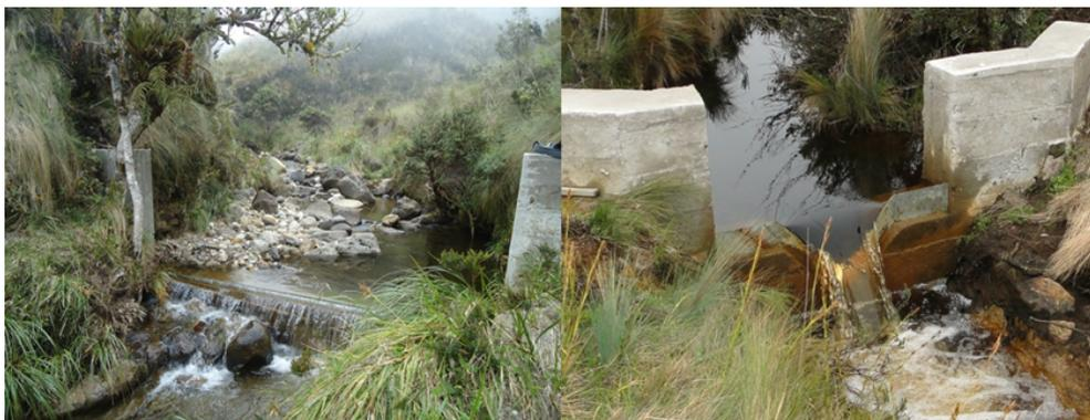
Figure 2. Examples of a rectangular weir (left) and a compound (V-notch-rectangular) weir (right) in the study area.
